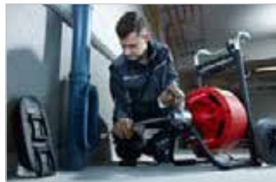
Cleaning of a down pipe with 16 mm spiral
