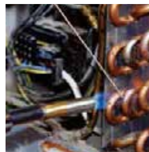
Brazing in refrigeration / air-conditioning technology
