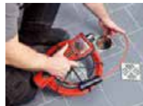
Inspection of floor drains
