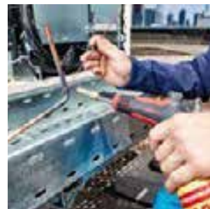
Brazing in refrigeration / air-conditioning technology
