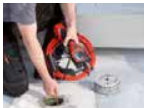
Inspection of rain downpipes
