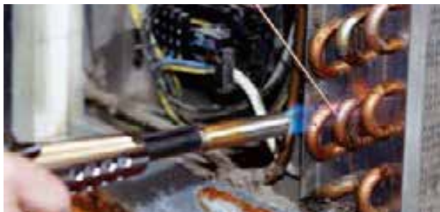
Brazing in refrigeration / air-conditioning technology
