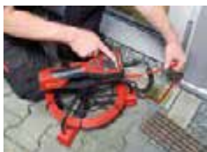
Inspection of rain drainpipes
