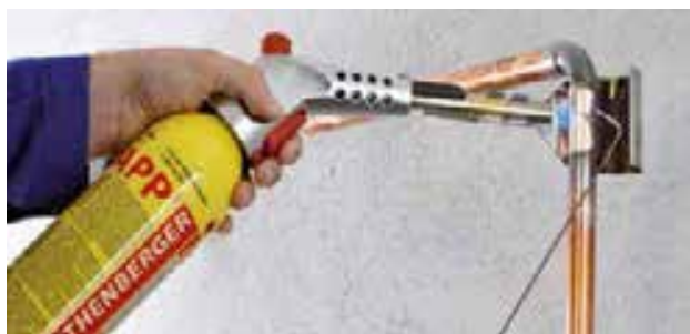
Brazing in gas installation
