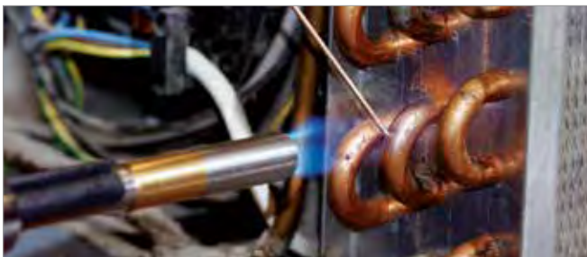
Brazing in refrigeration / air-conditioning technology
