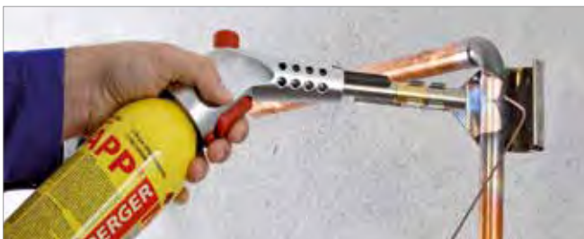
Brazing in gas installation
