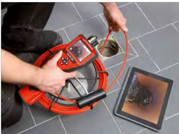
Inspection of basin drains
