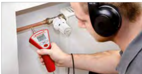
Acoustic leak detection of heating installations
