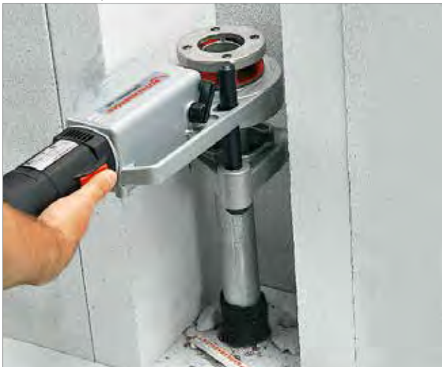
Work in confined spaces
