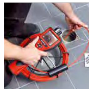
Inspection of floor drains
