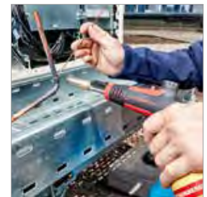
Brazing in refrigeration / air-conditioning technology
